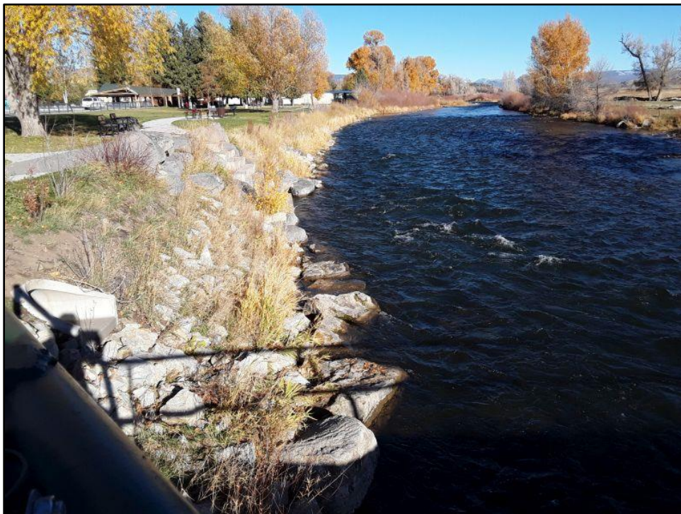
Photograph PH40. Overview of OHWM03 (White River), view facing east. Vegetation in riprap lacks dominant hydrophytic vegetation species.
